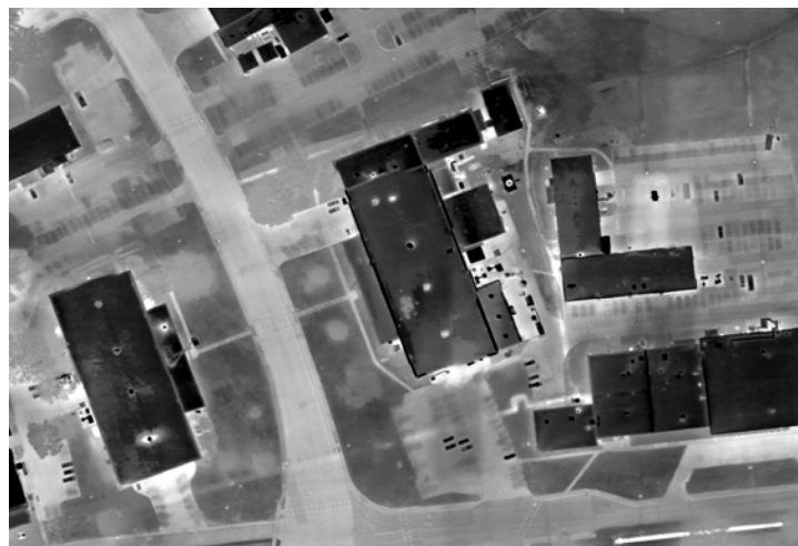
Thermal orthomosaic of a corporate campus showing pipes down to 2 meters underground.
